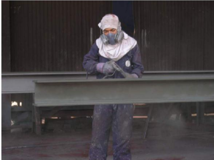
Application of primer immediately after abrasive blasting.
