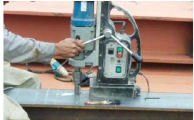
Drilling of bolt hole on I-section.
