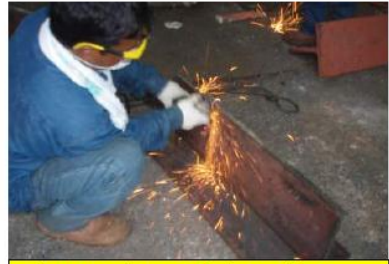
Edge grinding work for welding.
