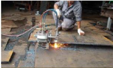
Cutting of steel plate by using mechanical guided flame cutter.
