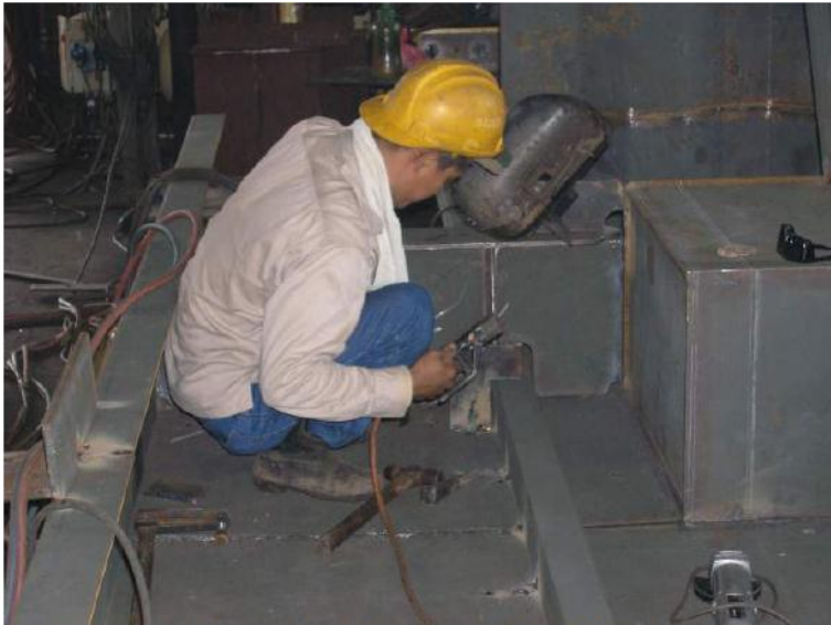
Manual Metal Arc Welding (MMAW)/ Shielded Metal Arc Welding (SMAW)
